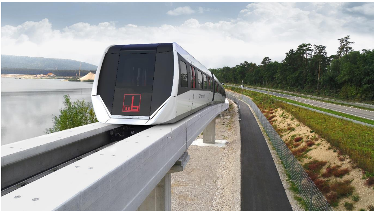
TSB on test track in Sengenthal, Germany. Credits: Firmengruppe Max Bögl
